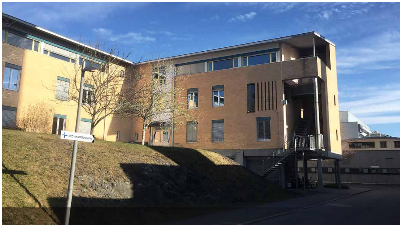
Akershus University Hospital, the emergency psychiatric department
