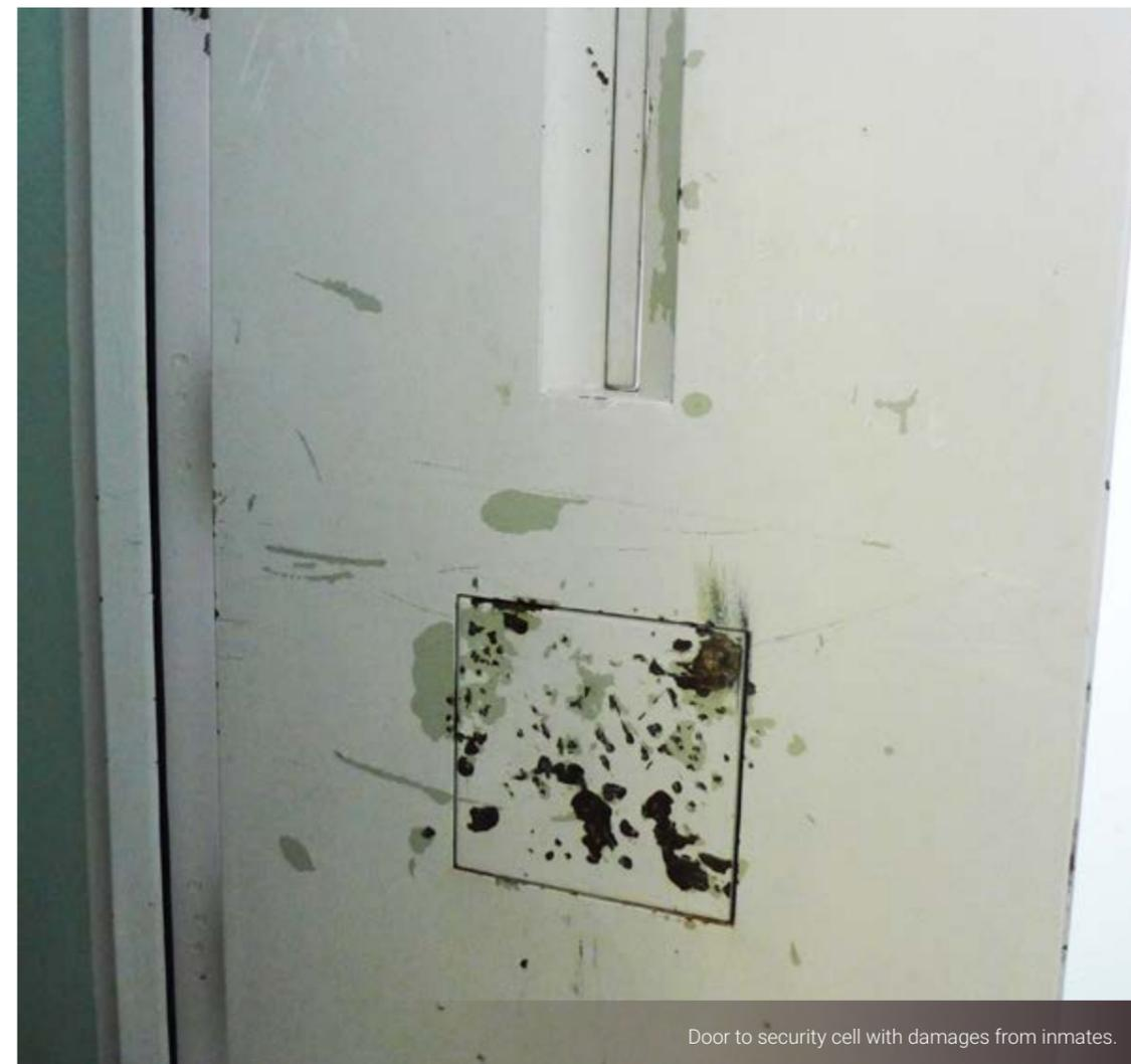
Door to security cell with damages from inmates.
